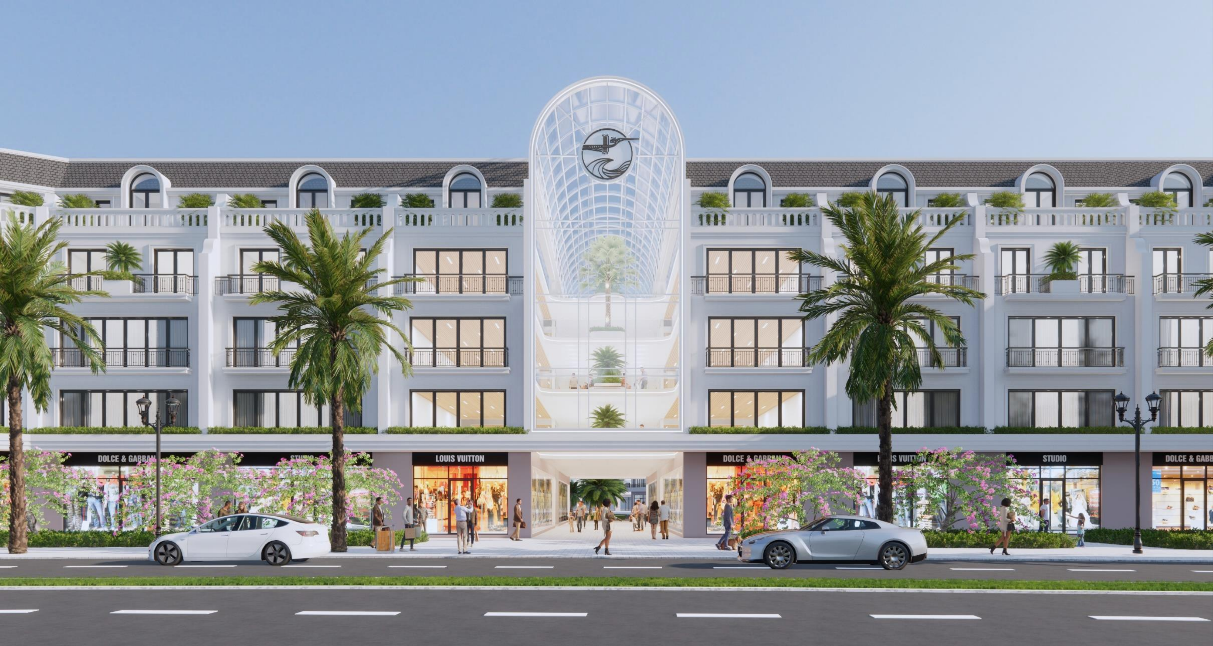
The façade means "Gateway to Heaven" with a large transparent glass panel that strongly contrasts the neighboring blocks.
